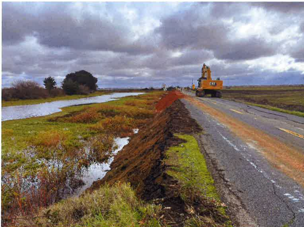
Re-establishing the waterside slope prior to placement of 18" minus riprap.
