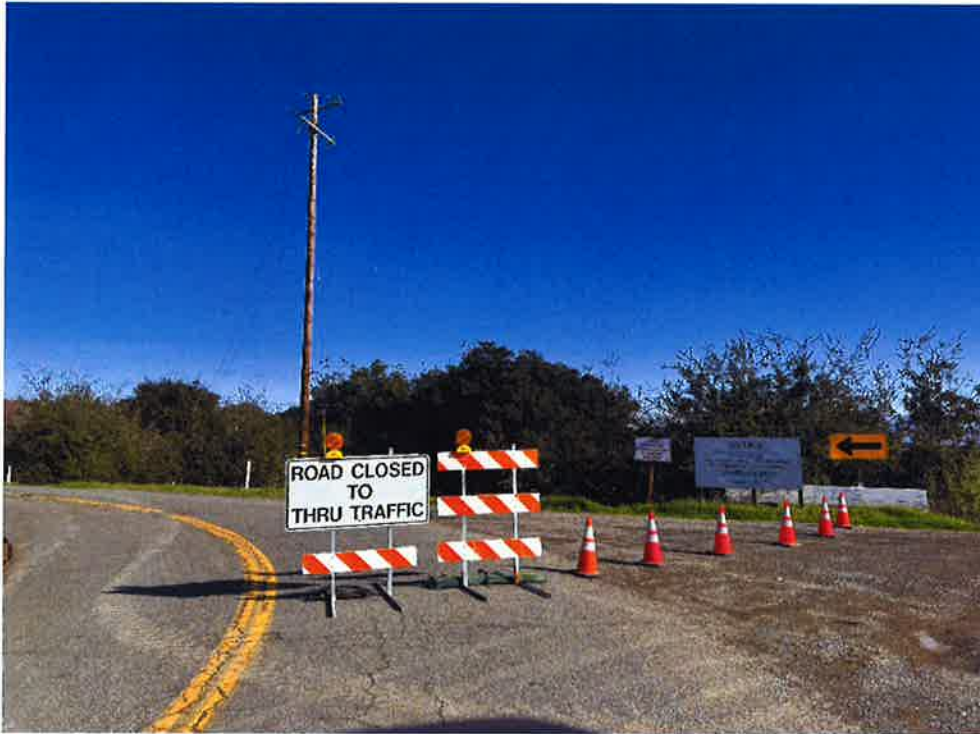
Traffic control at W. Brannan Island Road and Hwy 160 showing the westbound lane open to allow for outgoing trucks to return to the quarry for additional loads.
