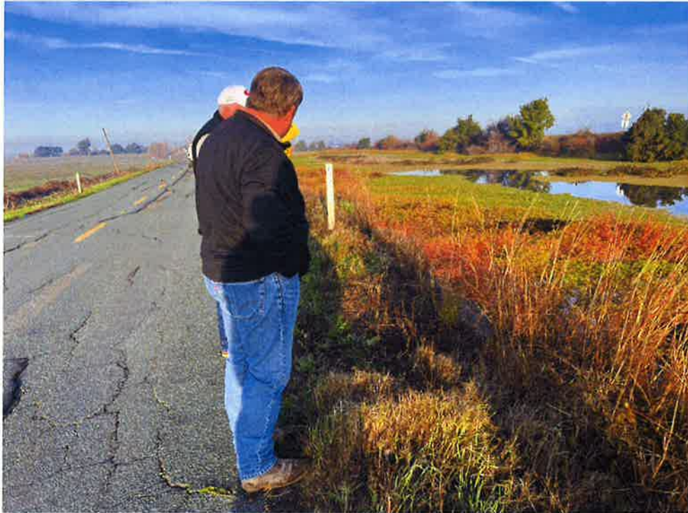
Twitchell Island Road near sta. 230+00 before the initiation of emergency work.
