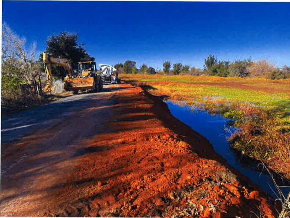
Re-establishing the Twitchell Island Road shoulder.
